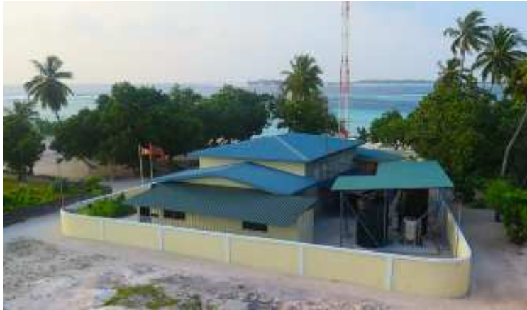
Power station in Gulhi island
